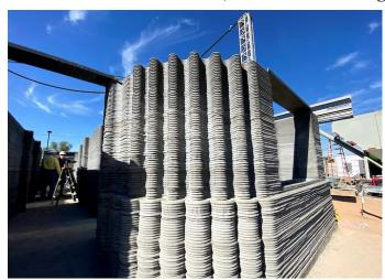
Figure 42: 3D printed exterior and interior walls, retained in their originally layered state
