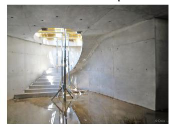
Figure 39: View of the stairs after removal of the 3D printed formwork
