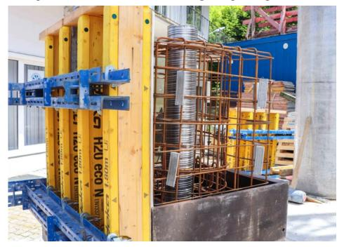
Figure 56: Complex formwork for concrete casting - 3D printing comes into action
