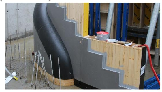
Figure 46: 3DP makes complex concrete formwork more efficient
